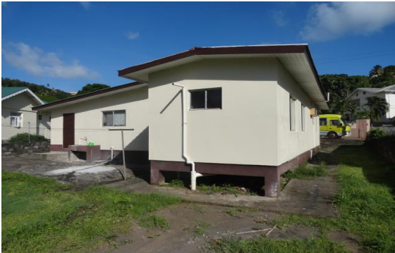
Side and rear view
